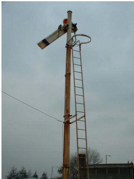
Semaphore at Redcliffe (Bascule) Bridge
